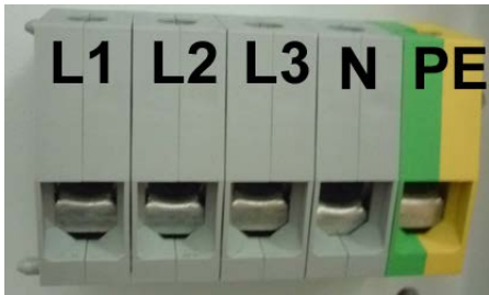
Fig. 17: Power Connection
